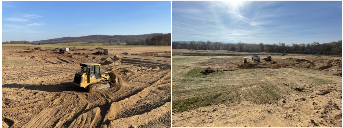
Work being done on a new wetland.
