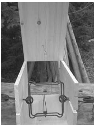
Body-gripping trap box during construction
